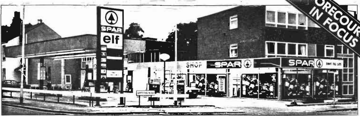
An Elf/Spar forecourt convenience store in South London.
