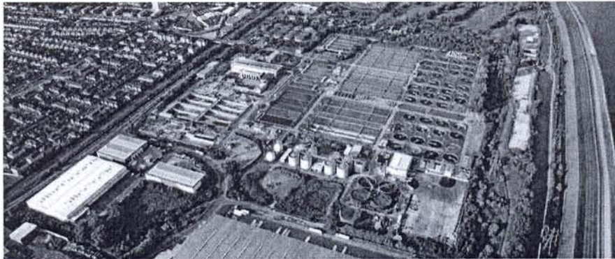
The upgrade will reduce odour from the works as well as improve local water quality
