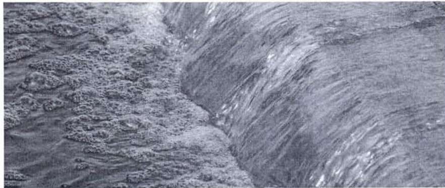
A full maintenance programme of all Severn Trent's assets is under way
